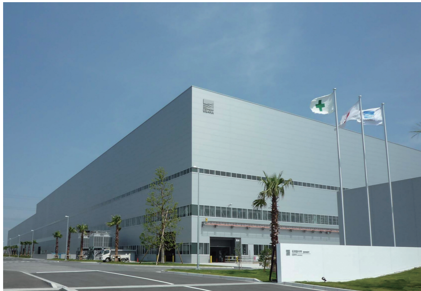
Ebara Corporation, Futtsu Plant
