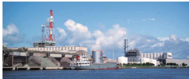
Liquid hydrogen power generation
