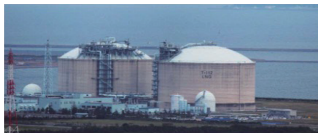
Liquid hydrogen receiving terminal
