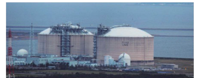
Liquid hydrogen receiving terminal
