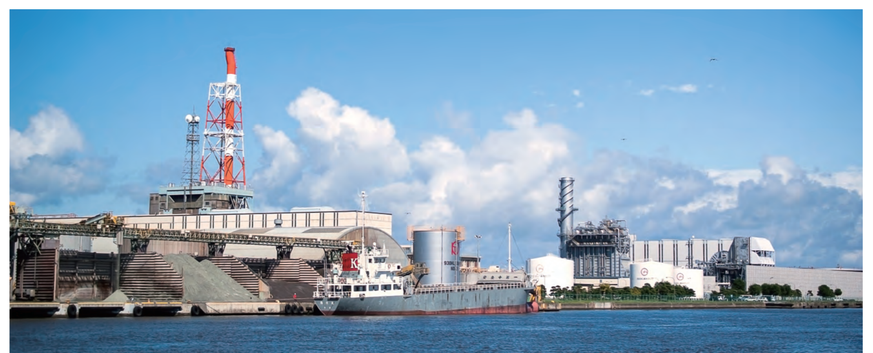
Liquid Hydrogen Power Generation
