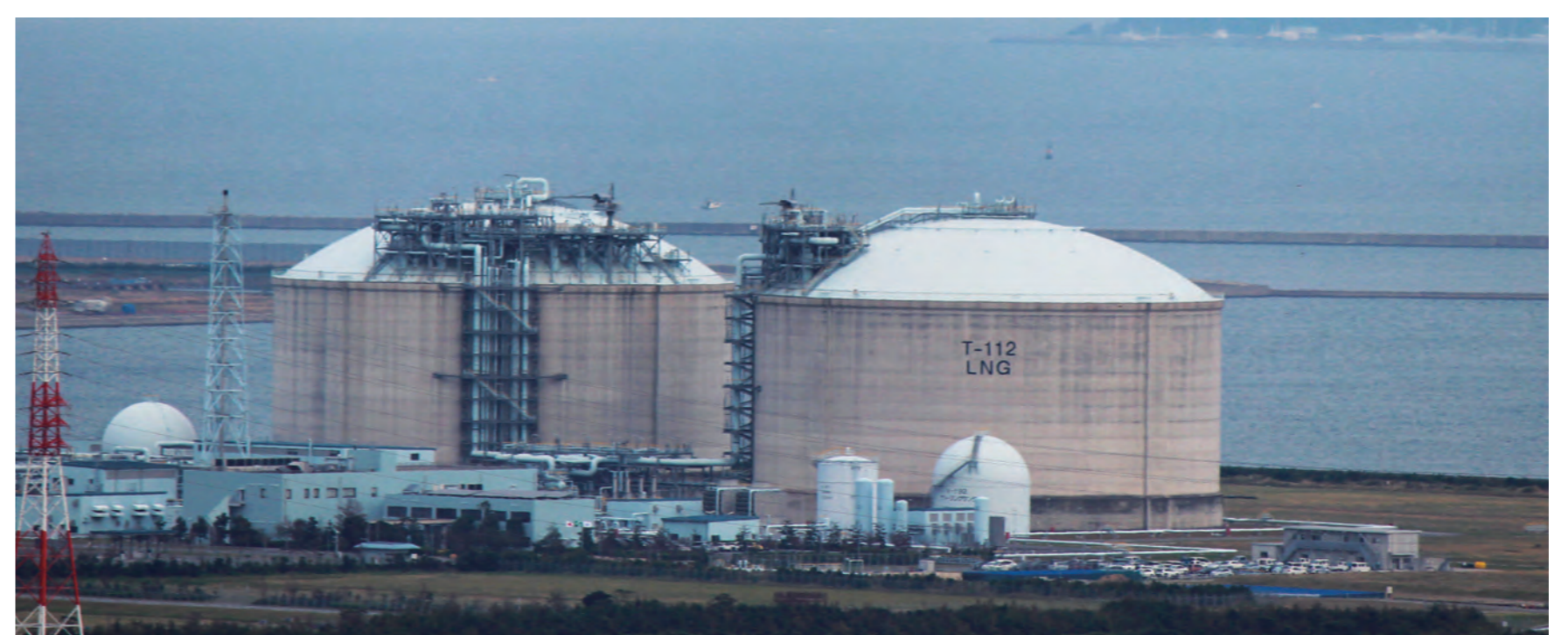
Liquid Hydrogen Receiving Terminal
