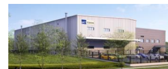
Image of completed overhaul base
