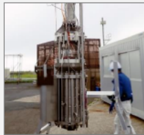
Liquid hydrogen booster pump
