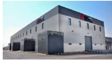
Photo of Saudi Arabia S&S site
