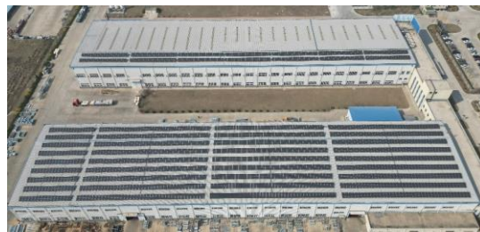
Solar power panels installed at Ebara Refrigeration Systems in China
