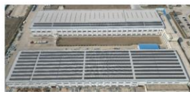
Solar power panels installed at Ebara Refrigeration Systems in China
