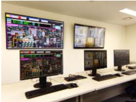
Remote support center
