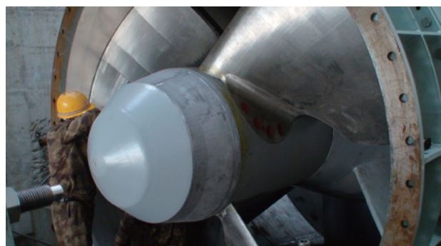
写真6 羽根車組立中 Photo 6 Assembly of the pump impeller
