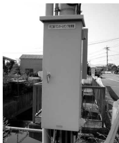
写真8 試験現場制御盤 (装柱型) Photo 8 Control board at field test site
