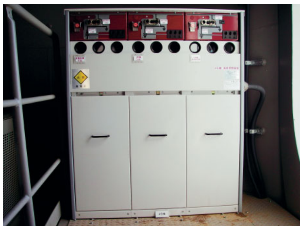
写真5 風車開閉器盤 (3面タイプ) Photo 5 Ring main unit (3 panel version)
