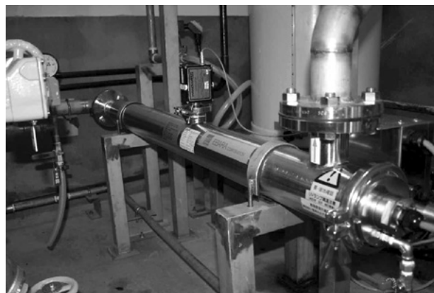
写真 納入紫外線照射装置 (AF3C-04-80W-2) Photo Delivered UV irradiation system
