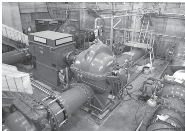
写真3 口径700 × 500 mm 横軸両吸込渦巻ポンプ Photo 3 Horizontal double-suction volute pump with 700 × 500 mm bore
