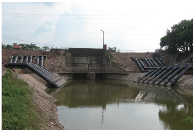
写真4 仮設緊急排水ポンプ場全景 Photo 4 Overview of temporary emergency drainage pumping station
