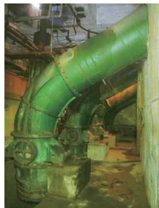
写真5 既設斜上吐出し立軸ポンプ Photo 5 Existing vertical pump with inclined discharge
