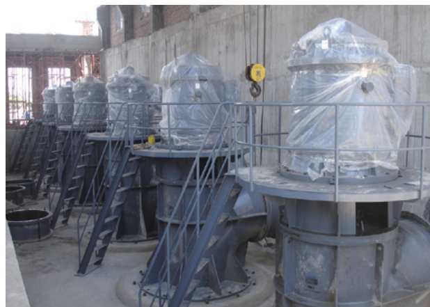
写真8 1床式立軸プルアウト式ポンプ（工事中） Photo 8 Pull-out type vertical pump with one floor arrangement (Under construction)
