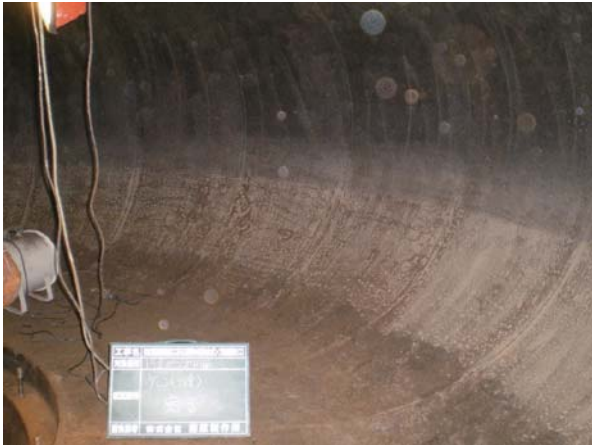
更新前 Before renovation
