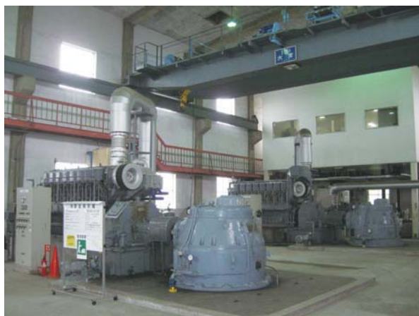
更新前 Before reconstruction
