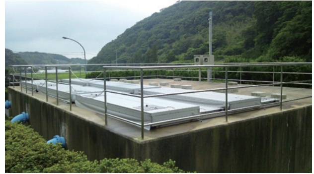
写真2 子々川浄水場活性炭吸着池 Photo 2 Granular activated carbon (GAC) adsorption filter in the Shishigawa water purification plant
